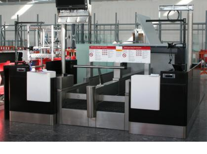
March 2007 was the start of the installation of 48 enclosures for the 'check in' desk in the arrivals hall at Terminal 5. The units consist of powder coated steel, stainless steel, interlayered glass and a range of specialist fittings conform to the rigid specifications required for airport construction.
